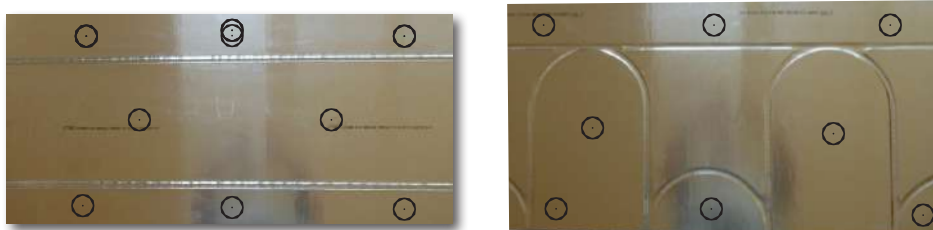
Install 8 anchors per board at the black dot locations as described above.
