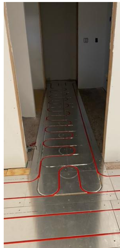
Above: Note the creative tubing layout designed to route tubing from the room down this narrow hallway.
